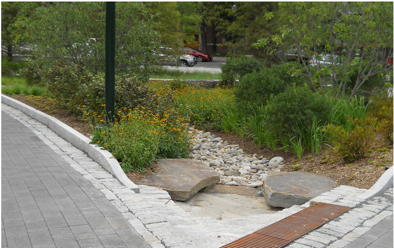
Green infrastructure best management practices (BMPs)—like this rain garden in Philadelphia, PA—utilize nature-based design to mitigate stormwater inundation and provide co-benefits such as improved water and air quality, wildlife habitation, and neighborhood beautification. BMPs contribute to sustainability and resiliency.
