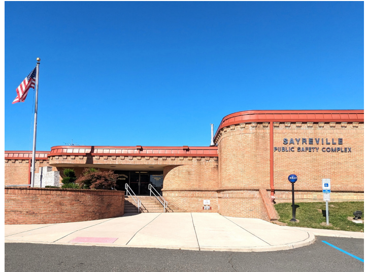
Sayreville Public Safety Complex
