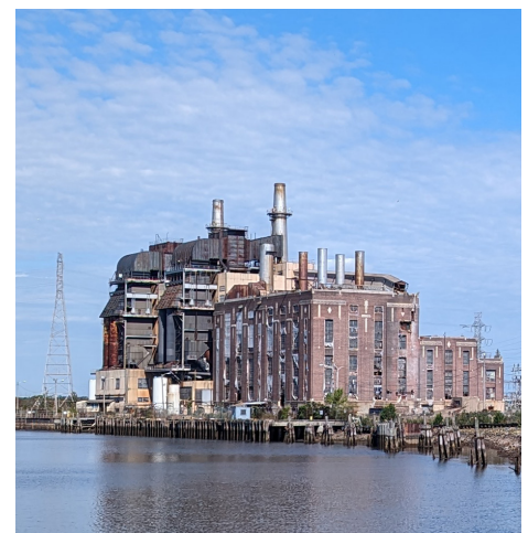
One of Sayreville's industrial sites along the Raritan River, located in the Borough's I District
