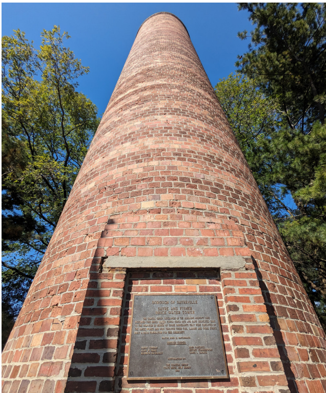
Sayre and Fisher Brick Water Tower
