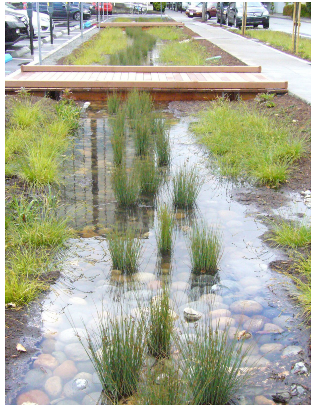
Rain garden in a parking lot in San Mateo County, CA Source: Flows to Bay, flowstobay.org
