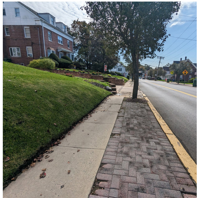
A portion of the sidewalk along Main Street
